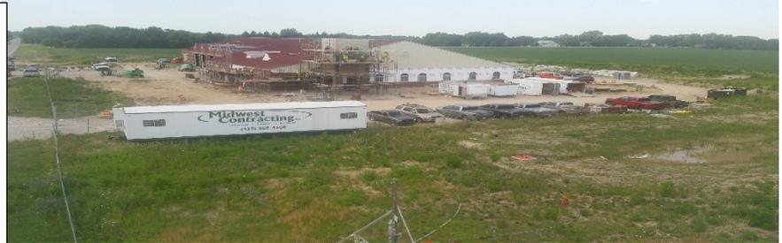
**UPDATES:** The roof is nearly completed. Nearly all of the windows are in. The dry wall is installed and is being finished. The floor drains and underground utilities are installed in the apparatus floor and concrete will be poured next week. Everything is starting to come together!
